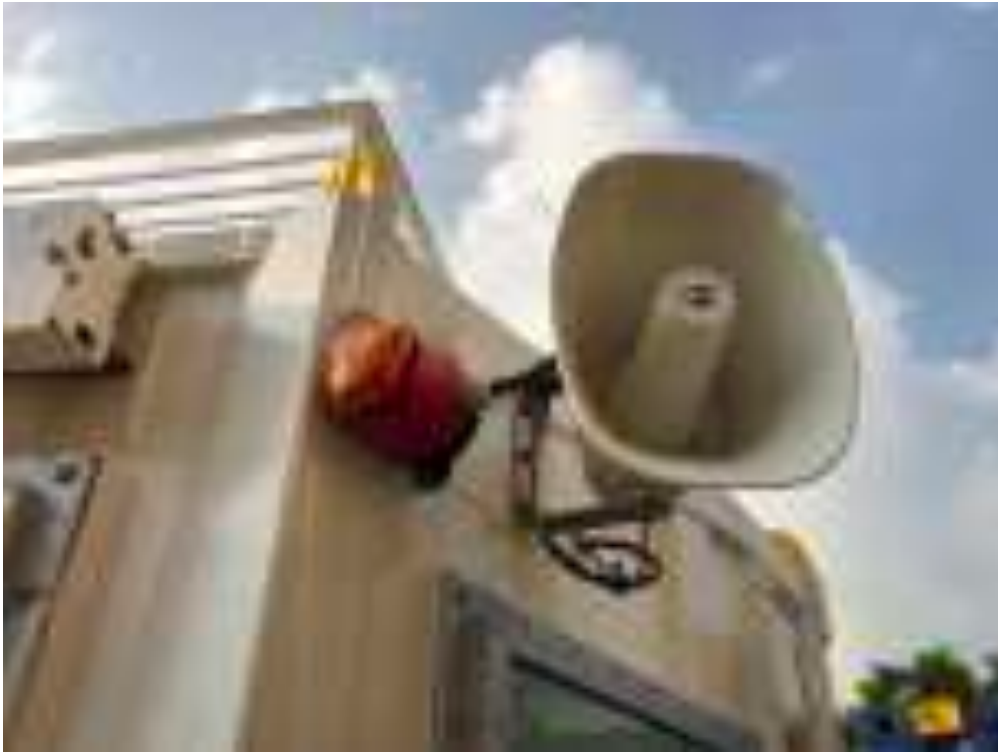
Gas Detector Strobe Light and Loud Speaker
